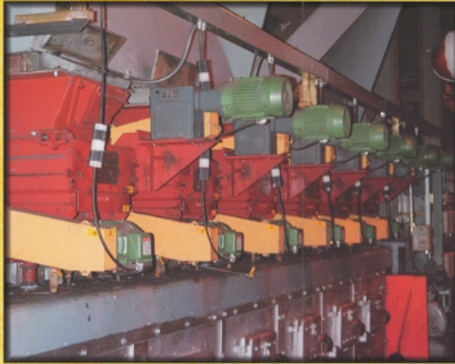
These Detroit® Underthrow Fuel Distributors feed coal at a municipal utility plant
