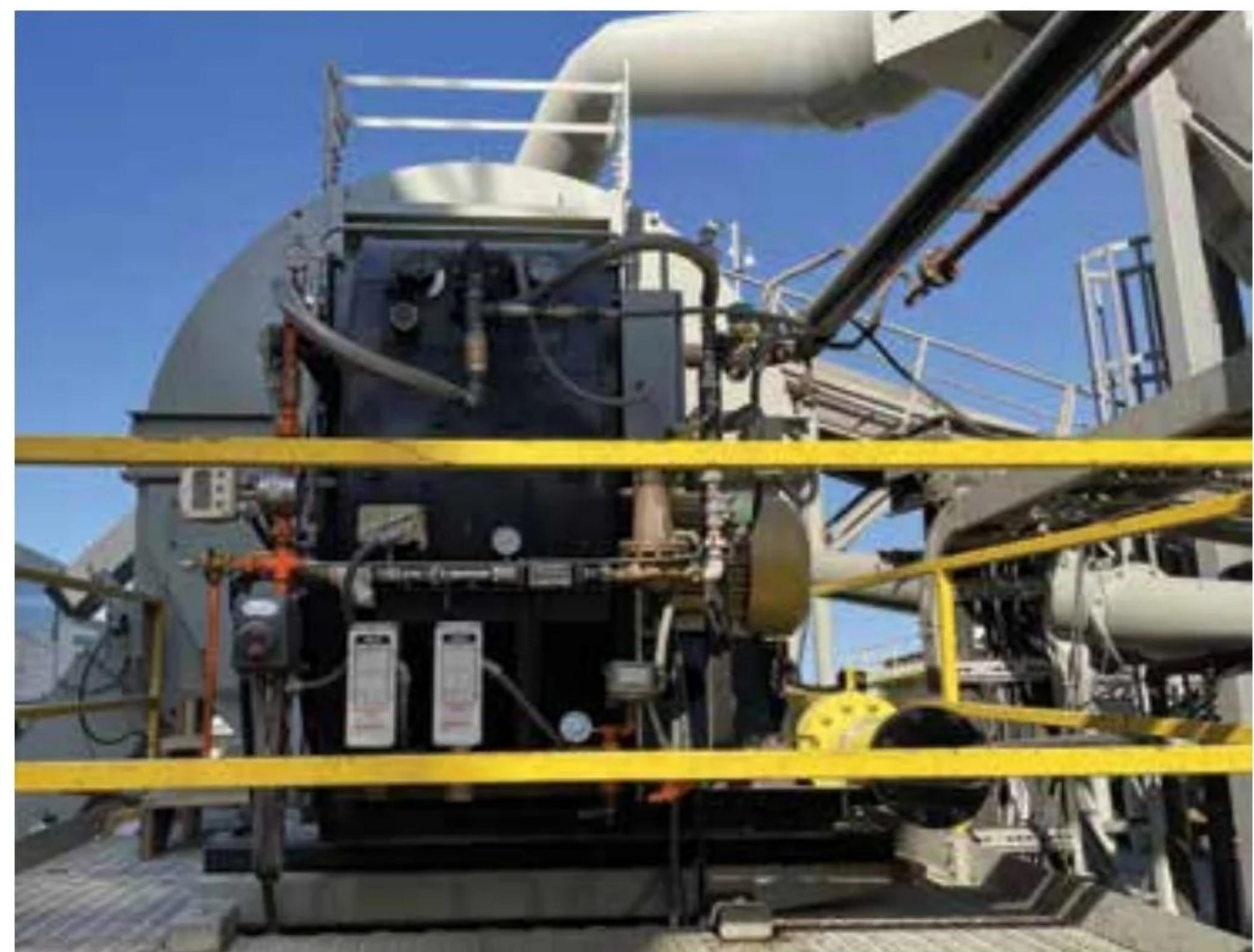
The David A. Bramble, Wye Mills, Maryland, burner replacement involved a comprehensive plant upgrade complete with new dryer, exhaust ducting, baghouse and exhaust fan. The old burner and the new light and waste oil fired Detroit HADES burner and HBC burner control panel are viewed from the burner end of the dryer in the photo above right.
