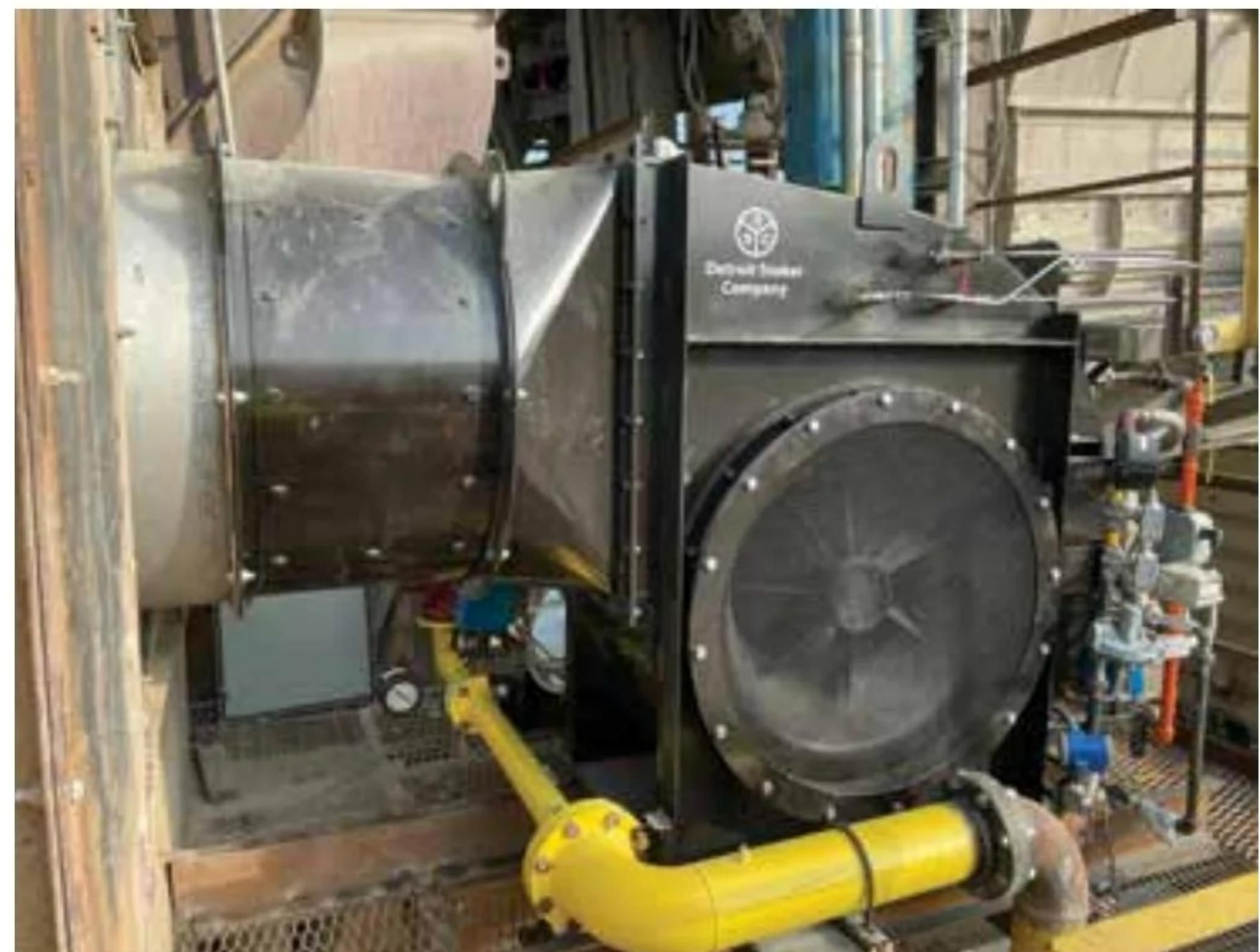
Eureka Stone in Milford, Pennsylvania, replaced its burner on a 2-ton batch plant. The burner fires on either compressed natural gas or No. 2 fuel oil. Here you can see the former open-fired burner replaced with a sealed in Detroit HADES burner. *All photos courtesy of Detroit Stoker Company Inc.*
